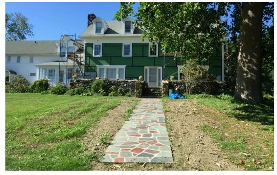
The slate/dirt walkway at the front of the main entrance has been removed and replaced with solid concrete, which was inlaid with the pieces of slate. The soil along the sides will be mulched or planted with grass.
